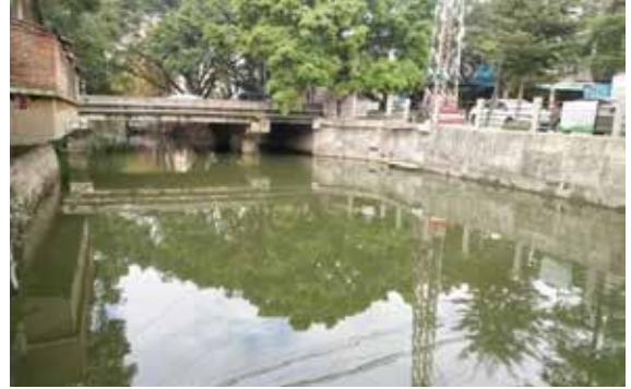
Black and odorous water after treatment 黑臭水體治理後
